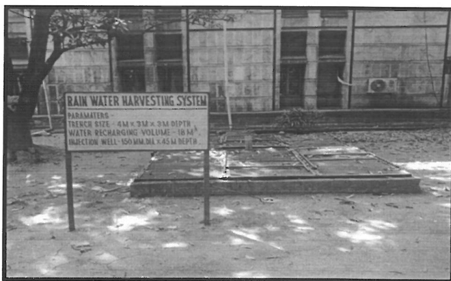
Photo- 18: Showing Rooftop Rain Water harvesting Structure
