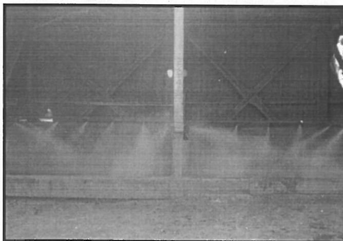
Photo: 6- Dry Fog Dust suppression system installed at under ground bunker & conveyors
