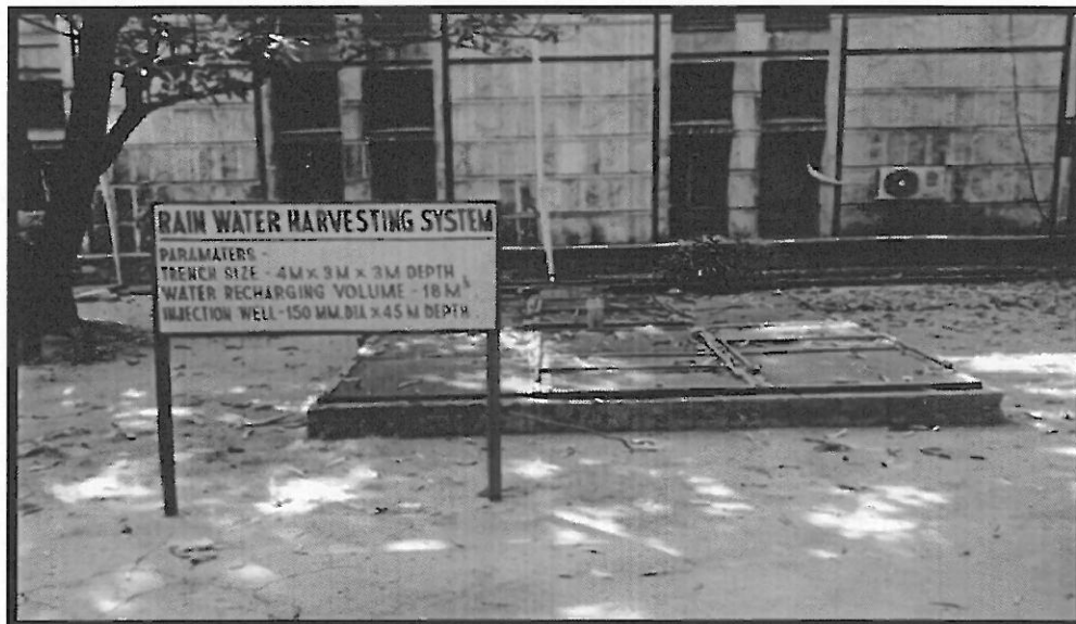
Photo-14: Rainwater Harvesting System
