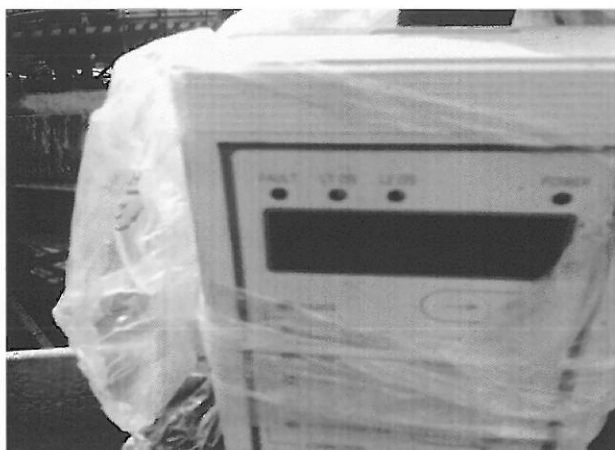
Photo-2 : Display unit of Online stack gas monitoring system attached to GCP stack of Furnace-1
