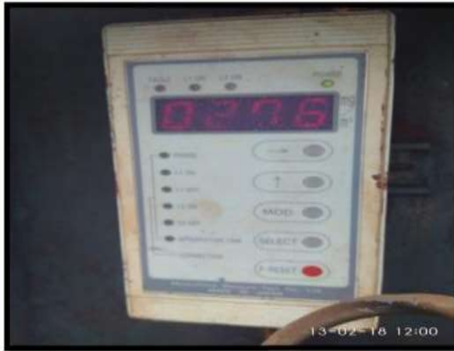
Photo-1: Showing Online Continuous stack monitor installed in the GCPstack attached to furnace
