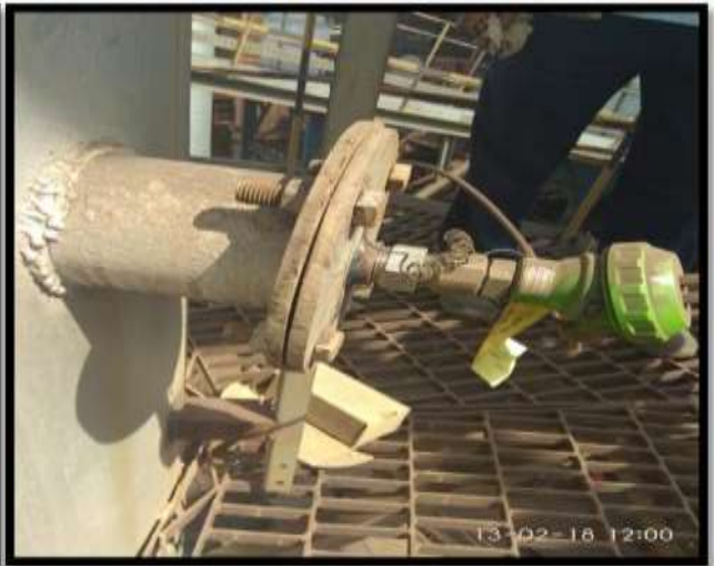
Photo-1: Showing Online Continuous stack monitor installed in the GCPstack attached to furnace
