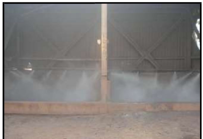
Photo:4- Dry Fog dust suppression system at screen house, underground bunker & conveyors
