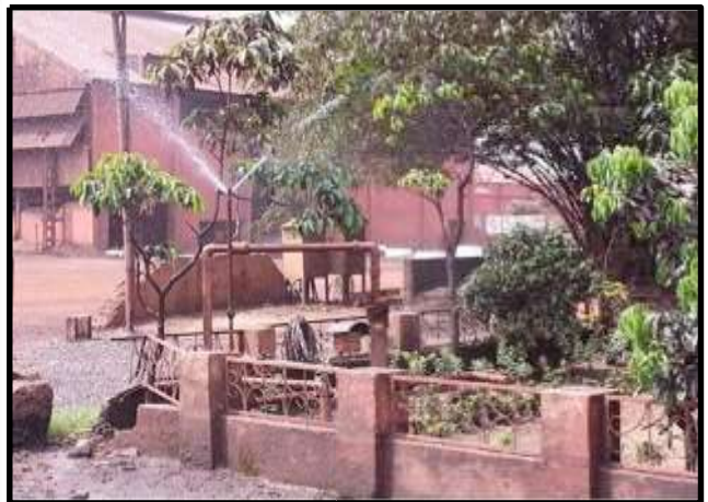
Photo: 3- Fixed Water sprinkling system
