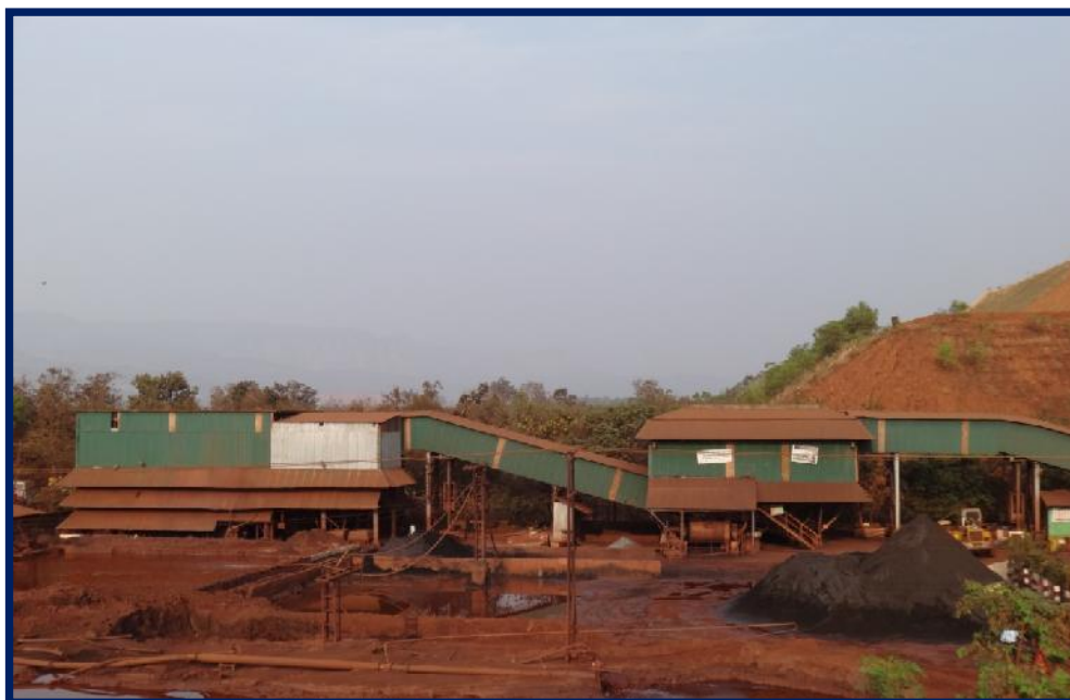
PHOTO-3 : SHOWING COB PLANT
