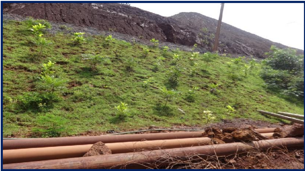
PHOTO-8: SHOWING COIR MATTING OVER DUMP SLOPE
