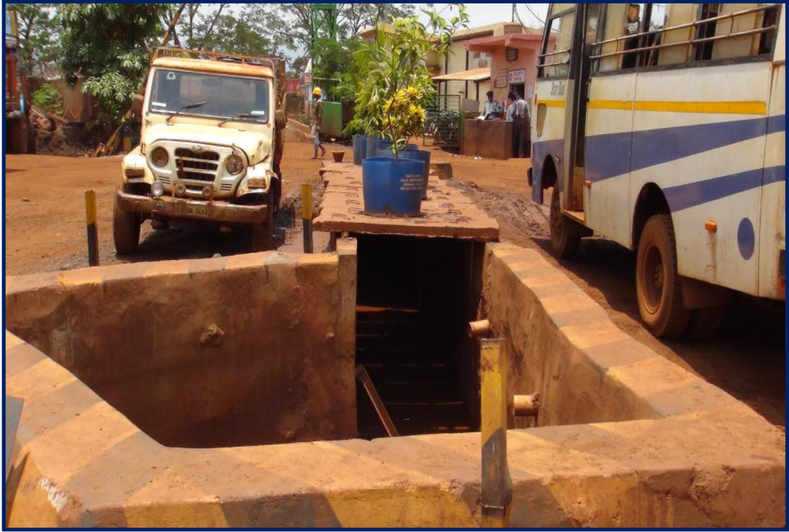
PHOTO-2: Showing concrete drain to channelize surface run-off to ETP through settling pit
