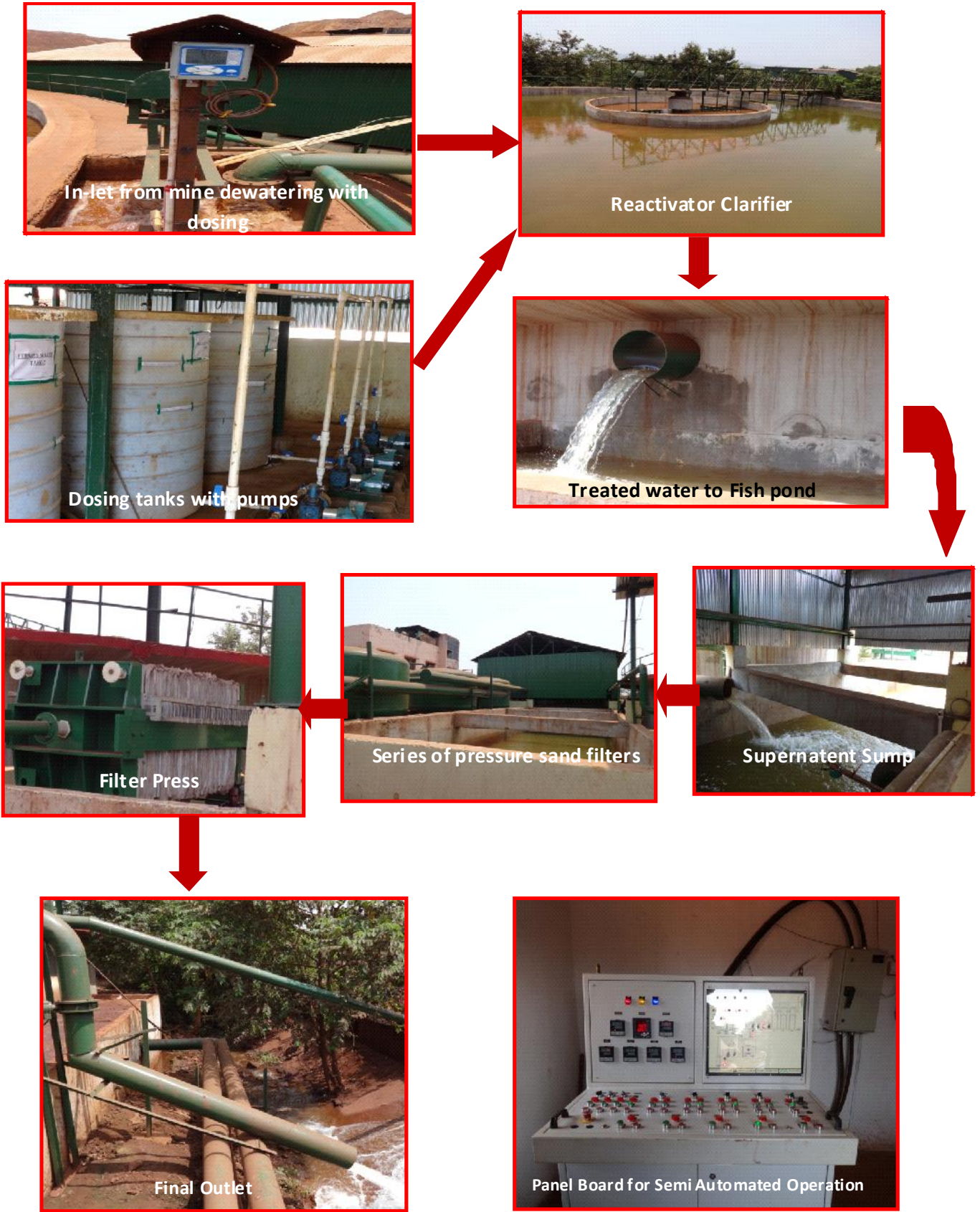
Figure-1: New up-graded ETP of capacity 445KL/Hr Process Flow Diagram
