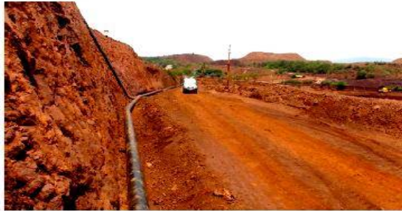
SURFACE RUN-OFF MANAGEMENT FROM TAILING POND AREA DUMP NO.- 03
