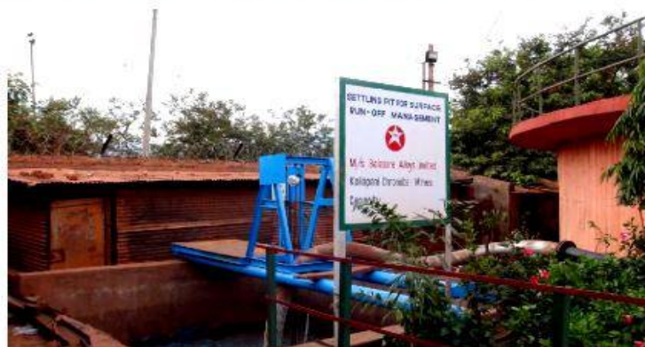
SURFACE RUN-OFF MANAGEMENT FROM COMMON DUMPING AREA TO ETP
