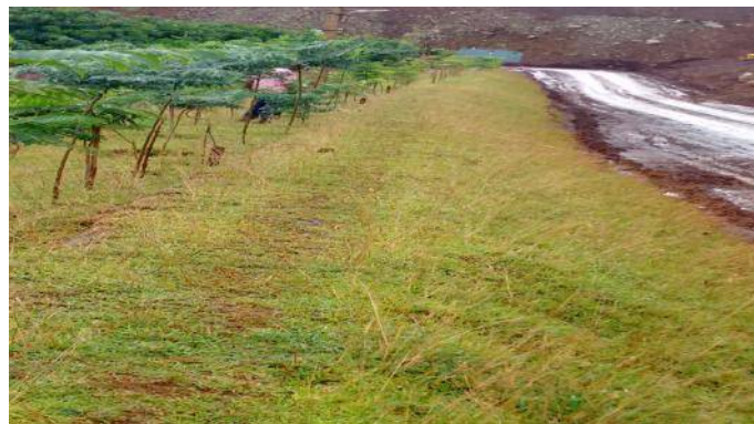
PHOTO-10: SHOWING GRASS TURFING OVER DUMP SLOPE
