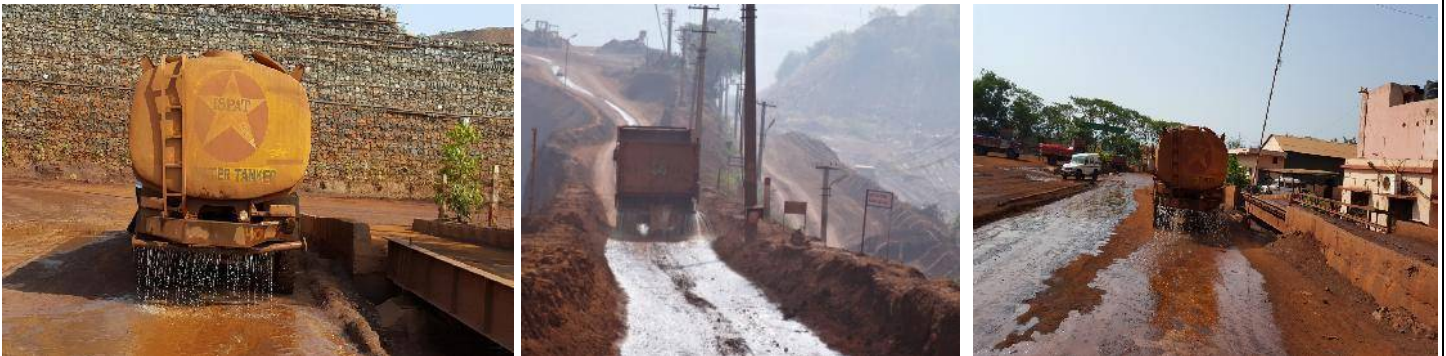
PHOTO-6 : SHOWING MOBILE SPRINKLERS INSIDE MINES
