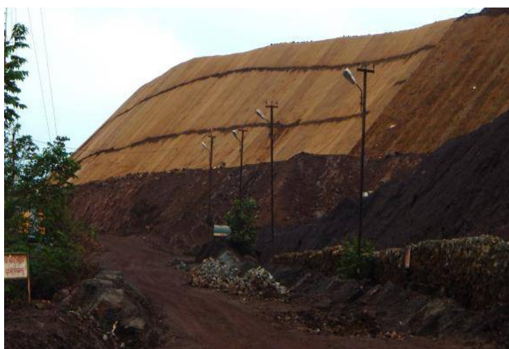
PHOTO-9: SHOWING COIR MATTING OVER DUMP SLOPE
