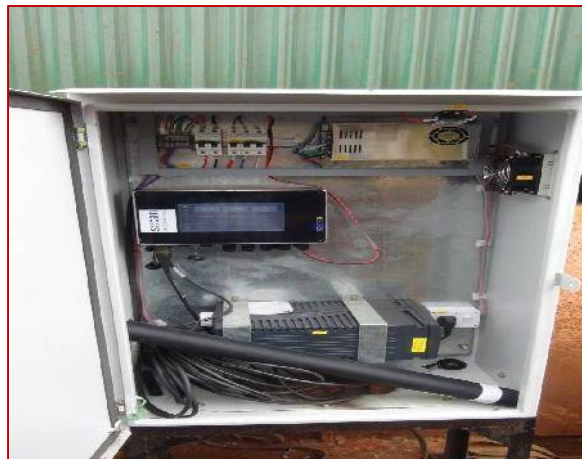
Photo-02: On-Line Monitoring System installed at In-let & Out-Let of ETP
