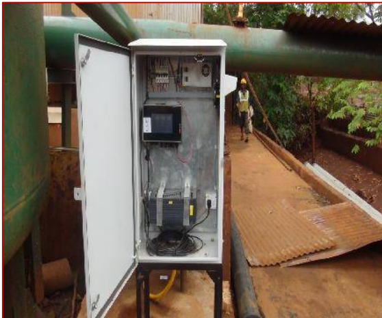
Photo-02: On-Line Monitoring System installed at In-let & Out-Let of ETP
