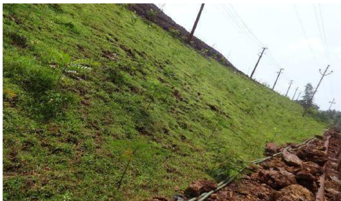
PHOTO-10: SHOWING GRASS TURFING OVER DUMP SLOPE
