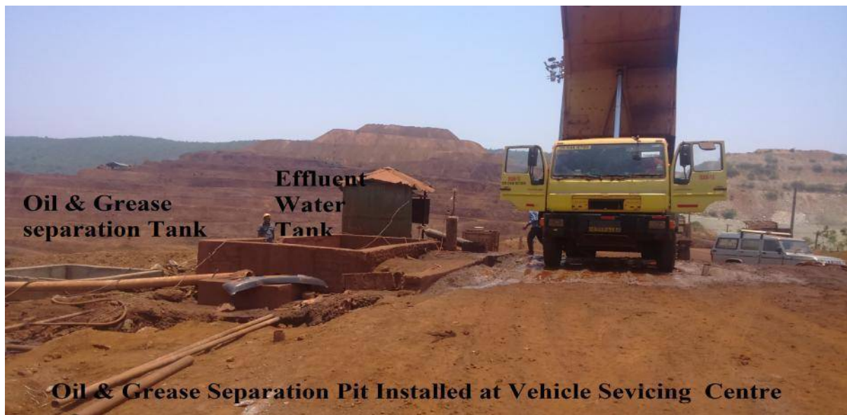
PHOTO-13: SHOWING VEHICLE SERVICING CENTER WITH OIL & GREASE TRAP
