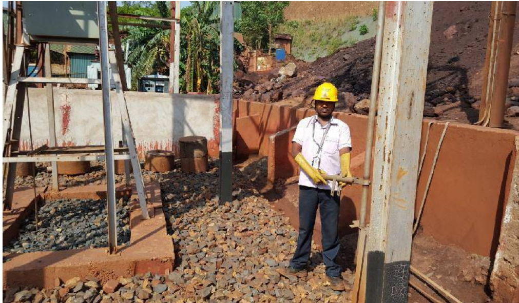
Photo-16: SHOWING WORKERS WORKING WITH PPE
