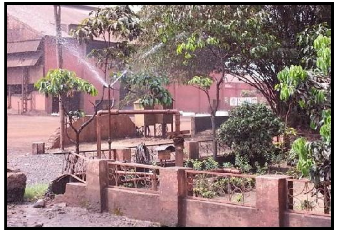
Photo: 4- Permanent Water sprinkling system
