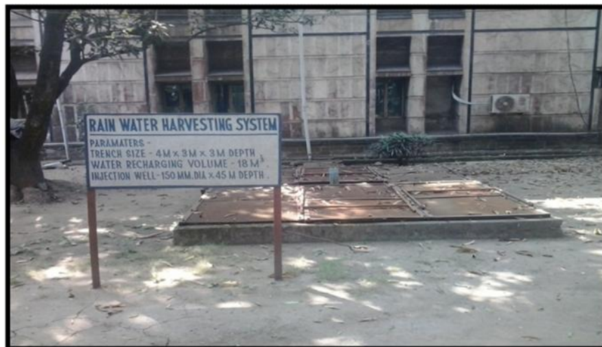
Photo- 18: Showing Rooftop Rain Water harvesting Structure
