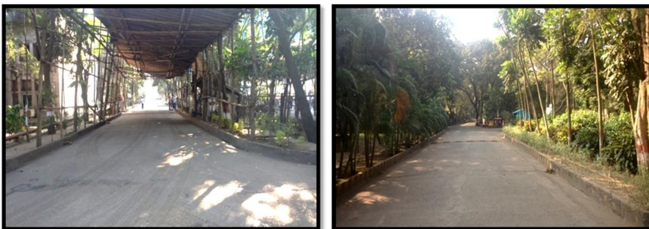
Photo-17: Showing Concrete haul roads inside plant premises
