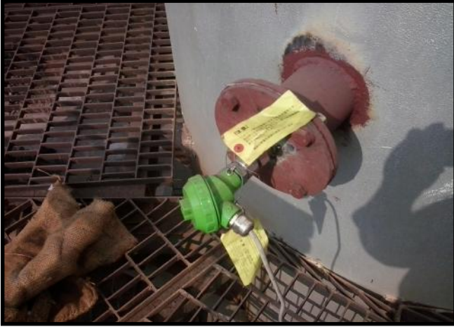
Photo-1 : Online stack gas monitoring system attached to GCP stack of Furnace
