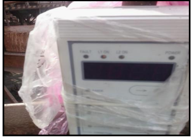
Photo-2 : Display unit of Online stack gas monitoring system attached to GCP stack of Furnace-1
