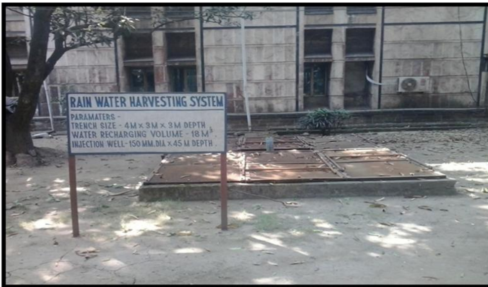
Photo-14: Rainwater Harvesting System
