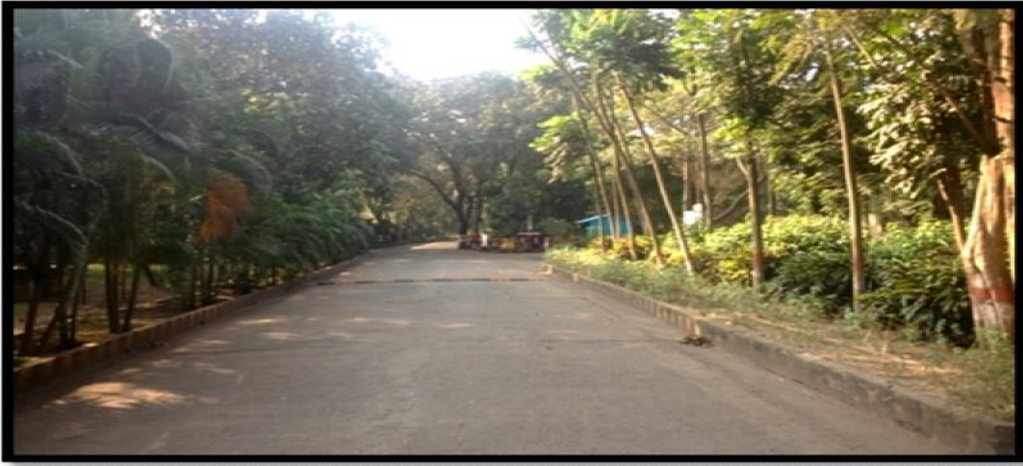
Photo-13: Concretion of Roads
