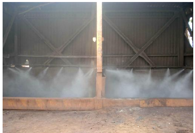
Photo: 6- Dry Fog Dust suppression system installed at underground bunker & conveyors
