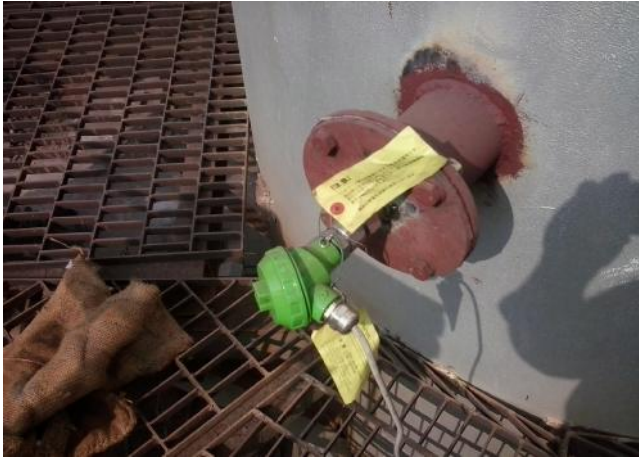
Photo-1 : Online stack gas monitoring system attached to GCP stack of Furnace-I
