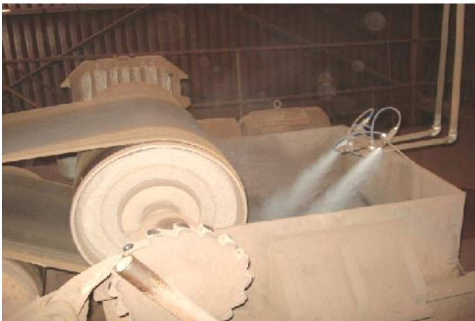
Photo:5- Dry Fog dust suppression system at screen house & transfer point
