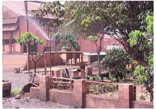
Photo: 4- Permanent Water sprinkling system
