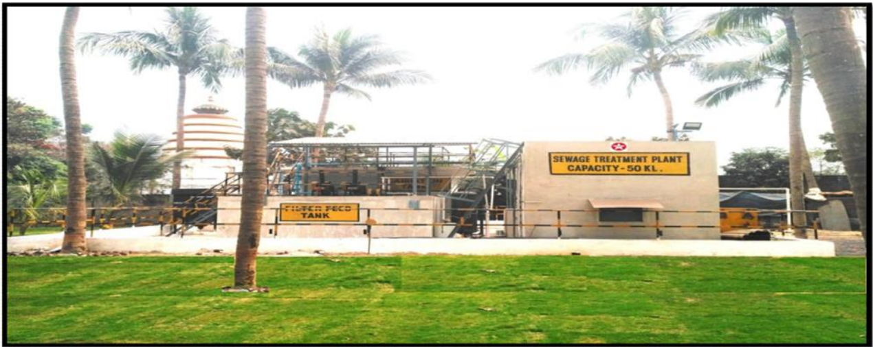
Photo: 9- Sewage Treatment Plant (STP) and treated water being reused in Horticulture & Dust Suppression
